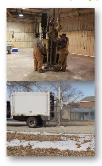
Phase II ESAs include soil and groundwater sampling – typically using direct push technology and laboratory analysis based on the RECs found in Phase I
